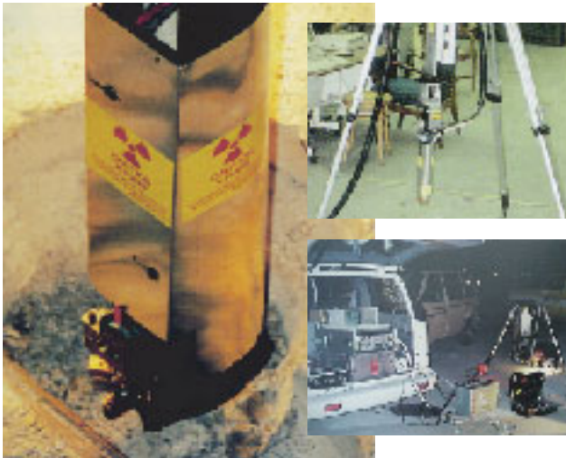
System to measure post-tensioning cables, LaGuardia Airport, N.Y.
