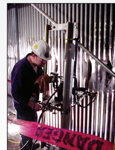
MEASURING RESIDUAL STRESS ON A RECOVERY BOILER
