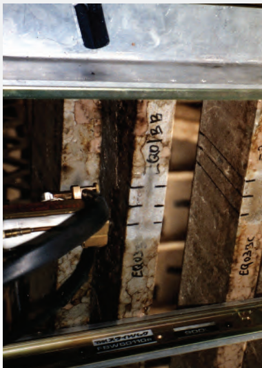
MEASURING DEAD LOAD ON EYEBARS OF FRANKLIN SQUARE BRIDGE
