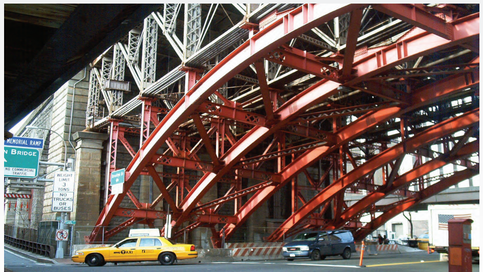
SUPPORT STRUCTURE ADDED TO FRANKLIN SQUARE BRIDGE
