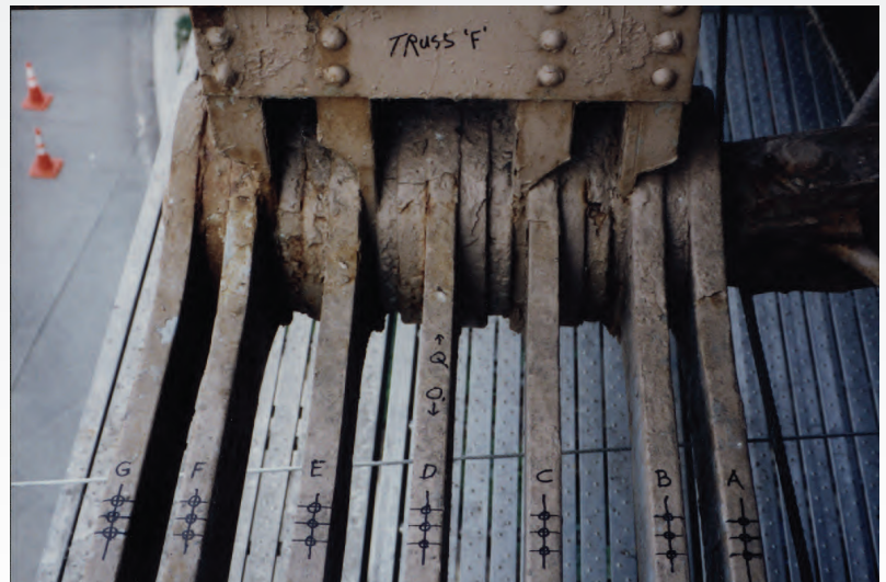
EYEBAR TRUSSES ON FRANKLIN SQUARE BRIDGE
