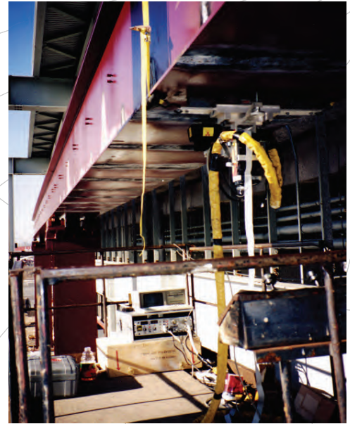
MEASURING DEAD STRESSES IN MONORAIL GIRDER
